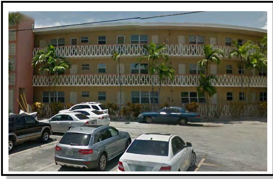
Photo No. 10: View of south adjoining property.
