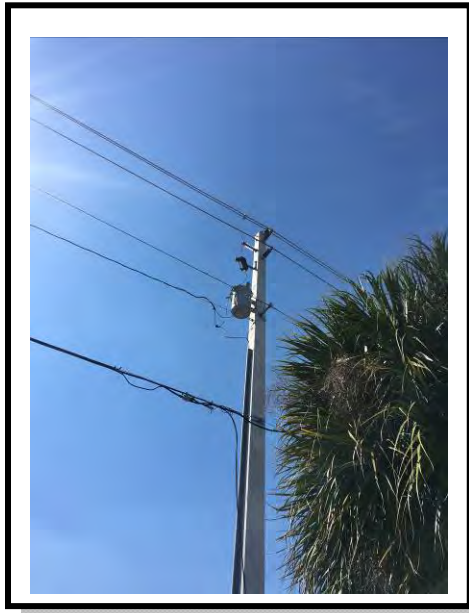
Photo No. 4: View of the pole mounted transformer.
