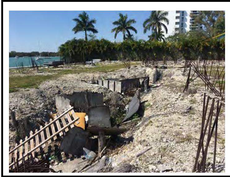
Photo No. 3: View of the dumped debris within the excavation area.
