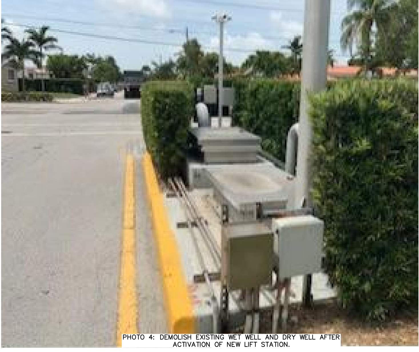
PHOTO 4: DEMOLISH EXISTING WET WELL AND DRY WELL AFTER ACTIVATION OF NEW LIFT STATION.
