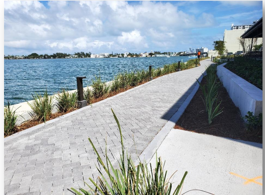
Benihana Island Walk & New Seawall
