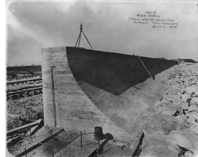
New seawall under construction in 1906, 15 feet high. (17 above low tide.)
