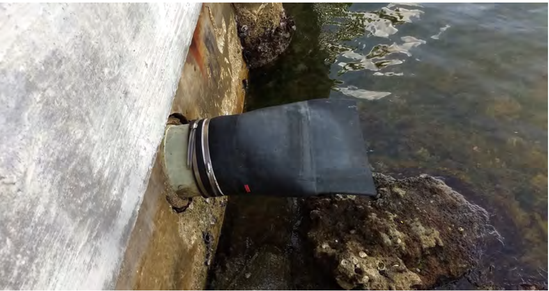
Backflow preventers installed at drainage outfalls in NBV. Photos and plans courtesy of NBV Public Works.
