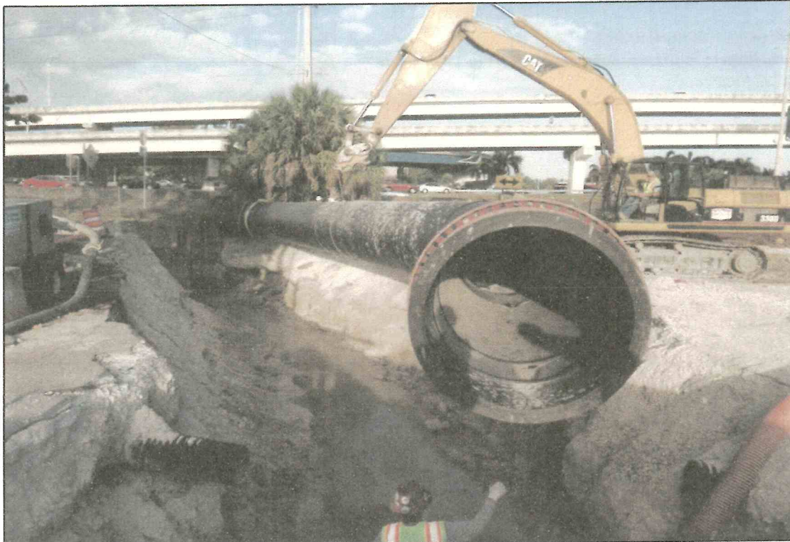
FIGURE 1: REPLACEMENT/REHABILITATION OF 72" FORCE MAIN (2016)
