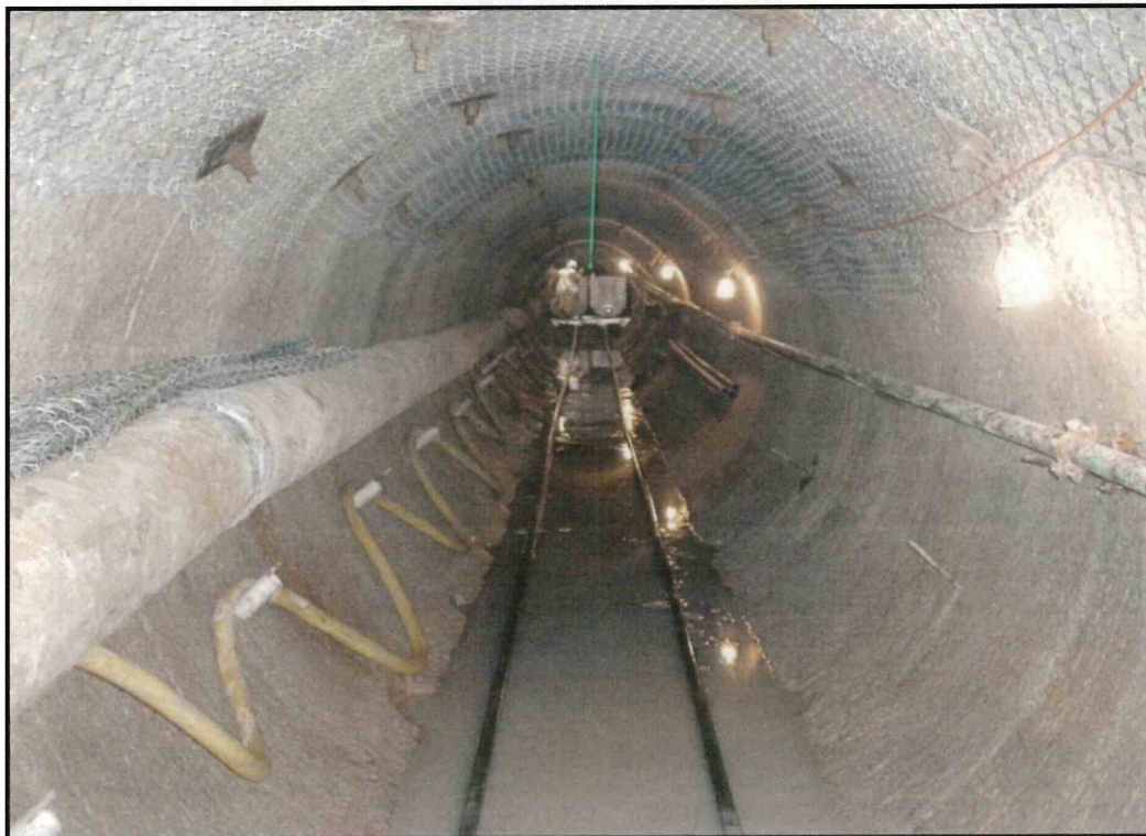
FIGURE 7: 48" PCCP GROUDED IN PLACE (CONTRACT B)
