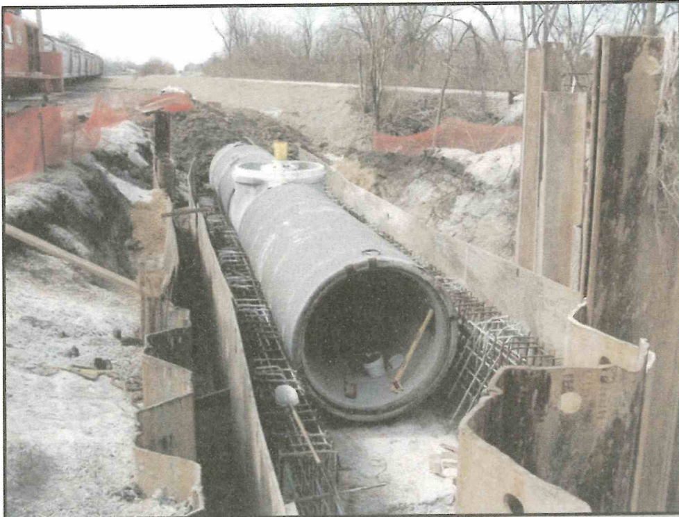
FIGURE 8: 66" PCCP WITH CONCRETE CRADLE
