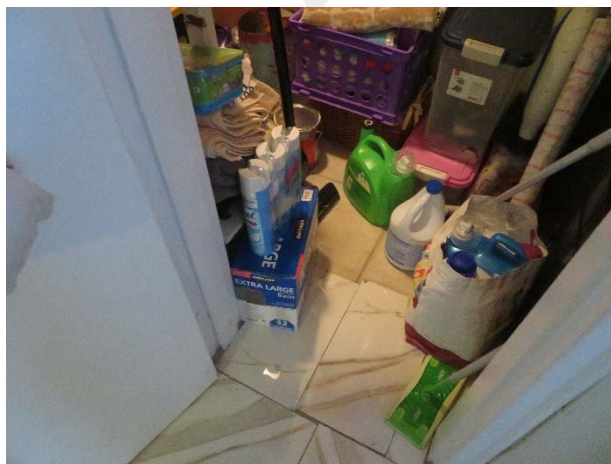
Figure 6. Two layers of tile installed over wood decking (Unit 206).
