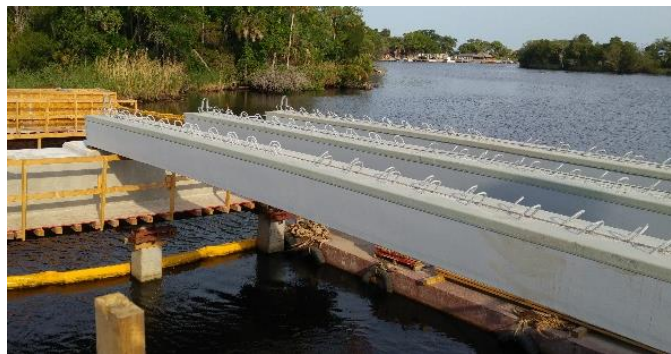
Figure 10. HCB during installation.
