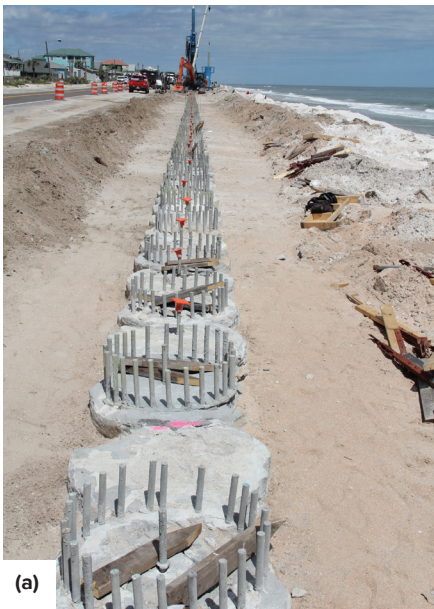
Fig. 7: After secant piles were installed: (a) the concrete guide wall was removed; (b) formwork and GFRP reinforcing bars were placed for the pile cap; and (c) a dune was constructed over the wall after the pile-cap concrete was placed and cured, and the pile-cap formwork was removed
