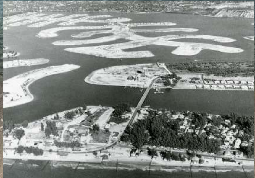
Dredging operations transformed Paradise Island and the Yacht Club Estates along the Treasure Island Causeway during the 1950s. (Image courtesy of Archives and Library, Heritage Village) [1]
