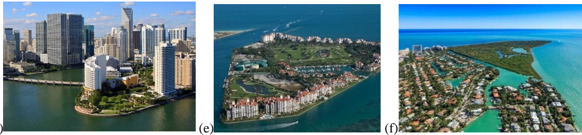
Fig. 5 Examples of RC seawall-bulkhead usage for land development on Florida's east coast: (a) Brickell Key, 1928 (b) Fisher Island, 1920's (c) Key Biscayne [1] , 1950's (d) Brickell Key [2] , 2011 (e) Fisher Island, 2015 (f) Key Biscayne, 2015.
