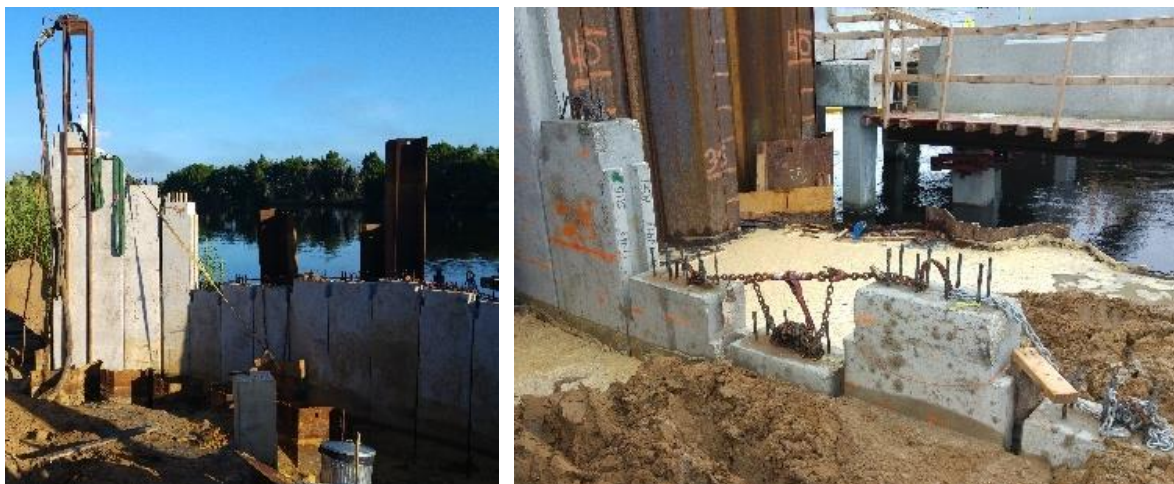
Figure 6. Sheet piles during installation
