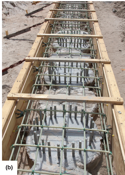
Fig. 7: After secant piles were installed: (a) the concrete guide wall was removed; (b) formwork and GFRP reinforcing bars were placed for the pile cap; and (c) a dune was constructed over the wall after the pile-cap concrete was placed and cured, and the pile-cap formwork was removed
