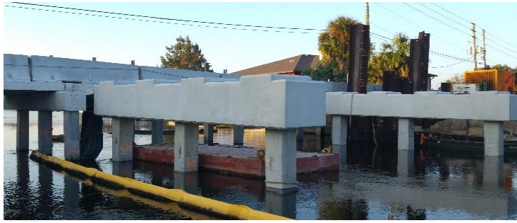
Figure 7. Pile bent cap after demolnding.
