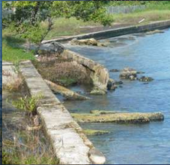
Cracking of existing seawall bulkhead cap
