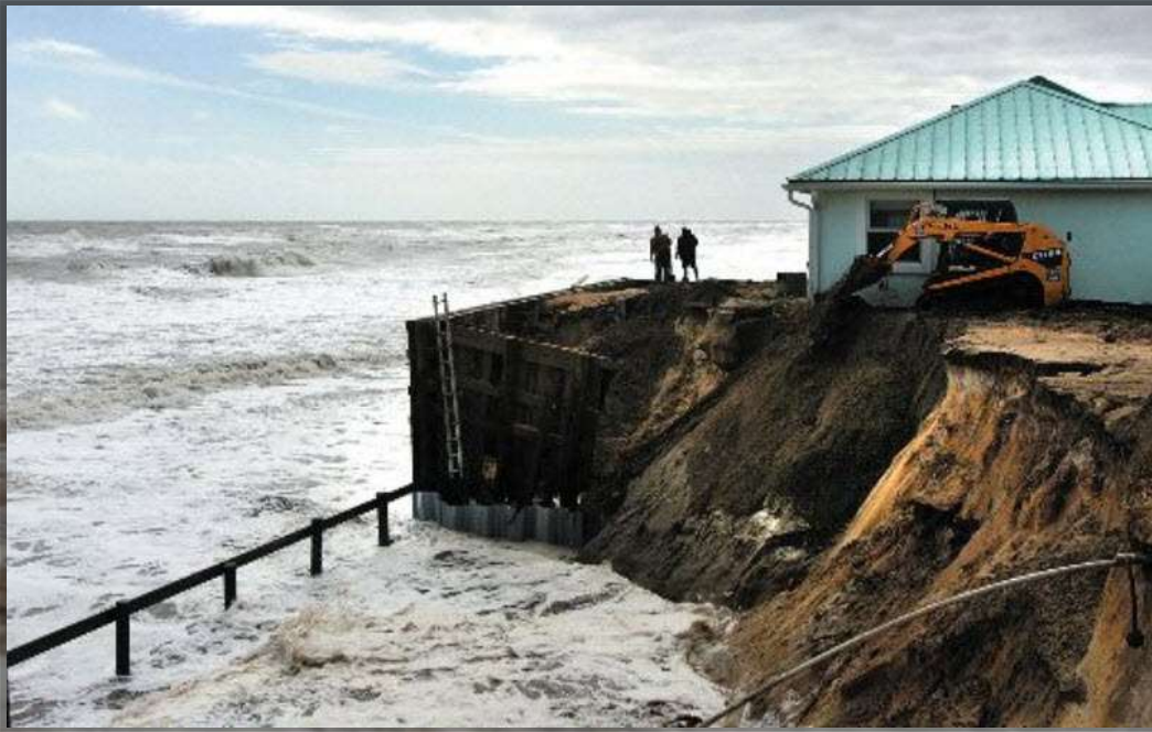
(a) Hurricane Damage along A1A (2008)
