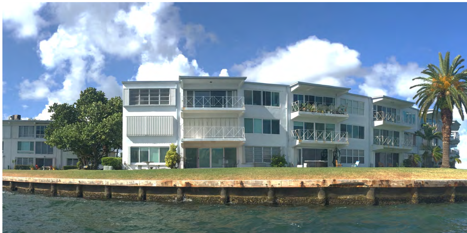
Current Condition of Seawalls
