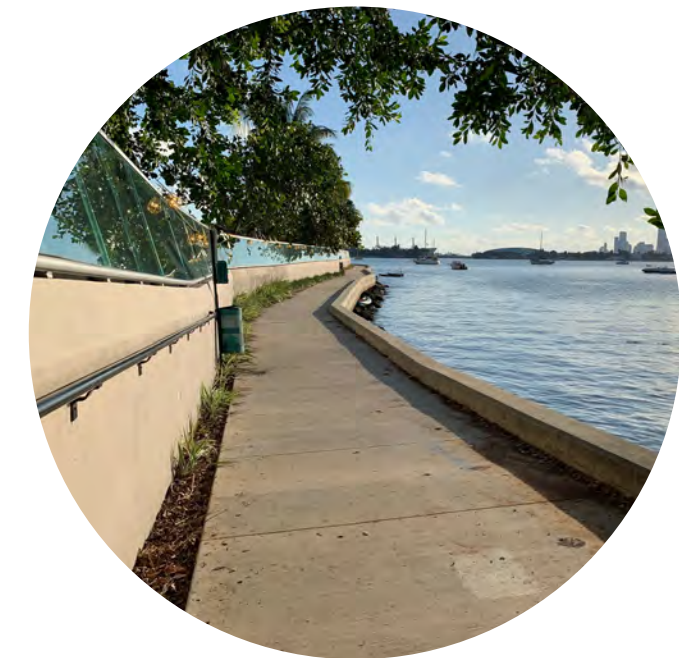
Biscayne Bay Path in Miami Beach features a narrow easement without adequate space for plantings and benches.
