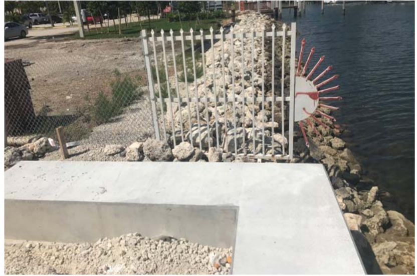
Figure 4-11: Typical Return Wall with Tie-rods and Concrete Cap Plan View and Photo
