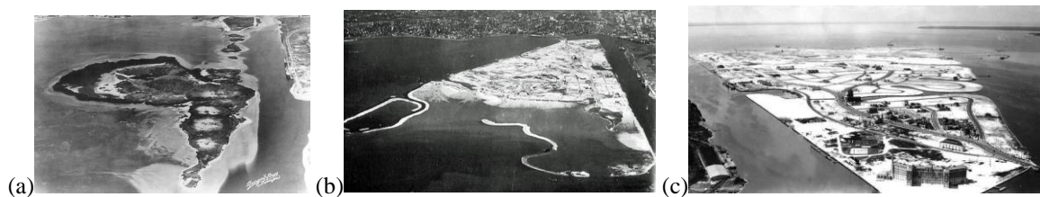
Fig. 7 Davis Island, Tampa Bay reclamation using RC seawall-bulkheads: (a) 1924; (b) 1925; (c) 1926. (Photographs courtesy of the Burgert Bros.)
