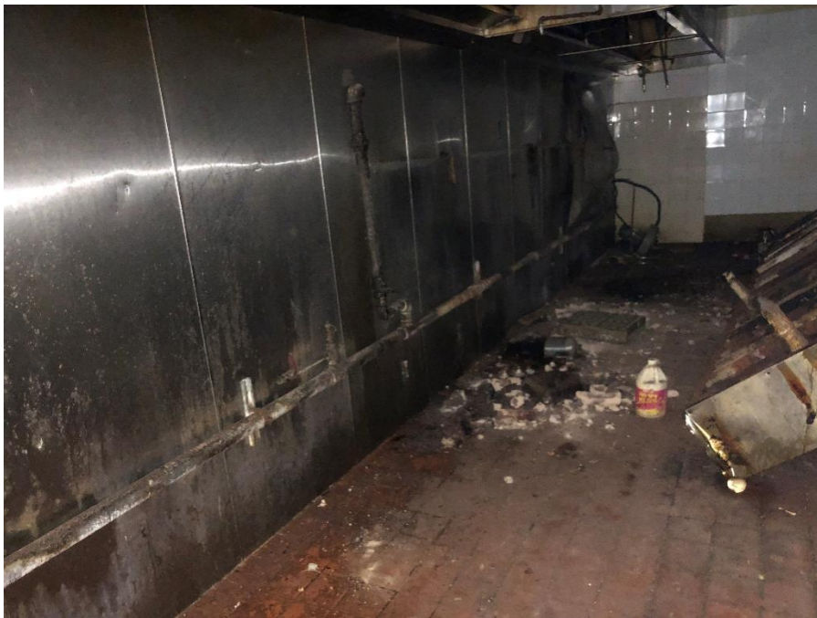
A typical view of the kitchen in the vacant restaurant.
