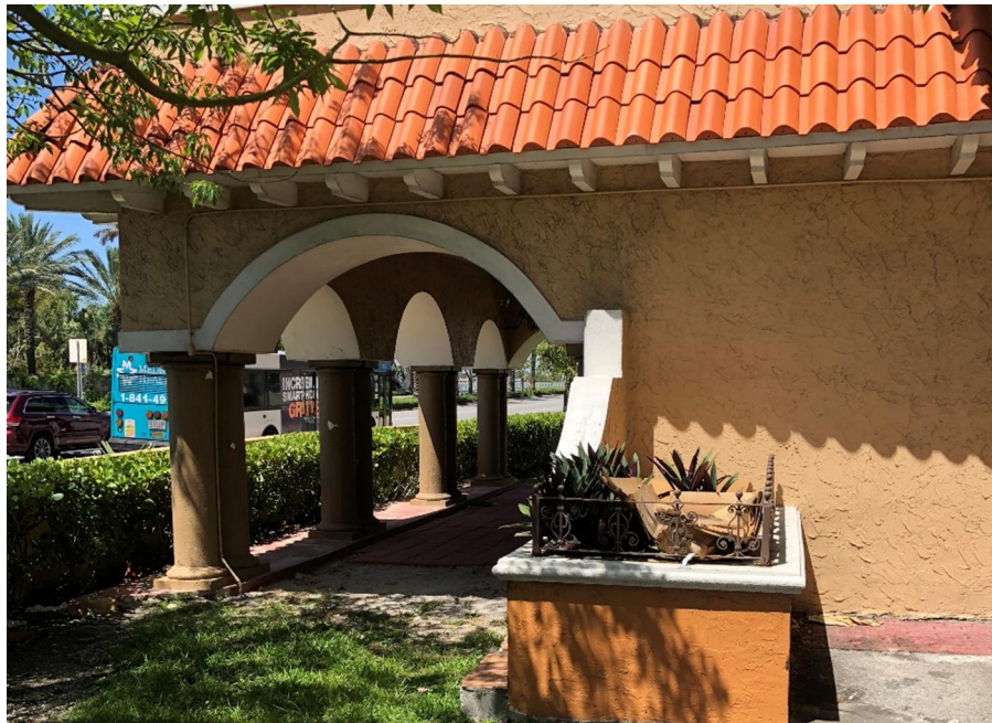
A view of the exterior of the subject property.
