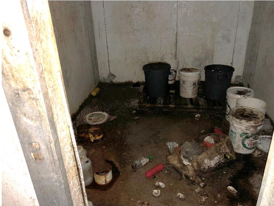
A typical view of the interior of the vacant restaurant.
