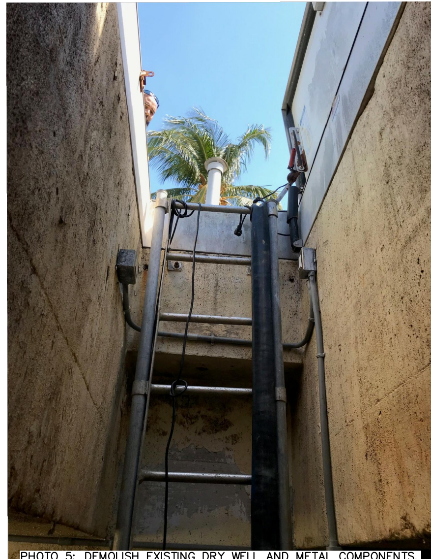
PHOTO 5: DEMOLISH EXISTING DRY WELL AND METAL COMPONENTS.
