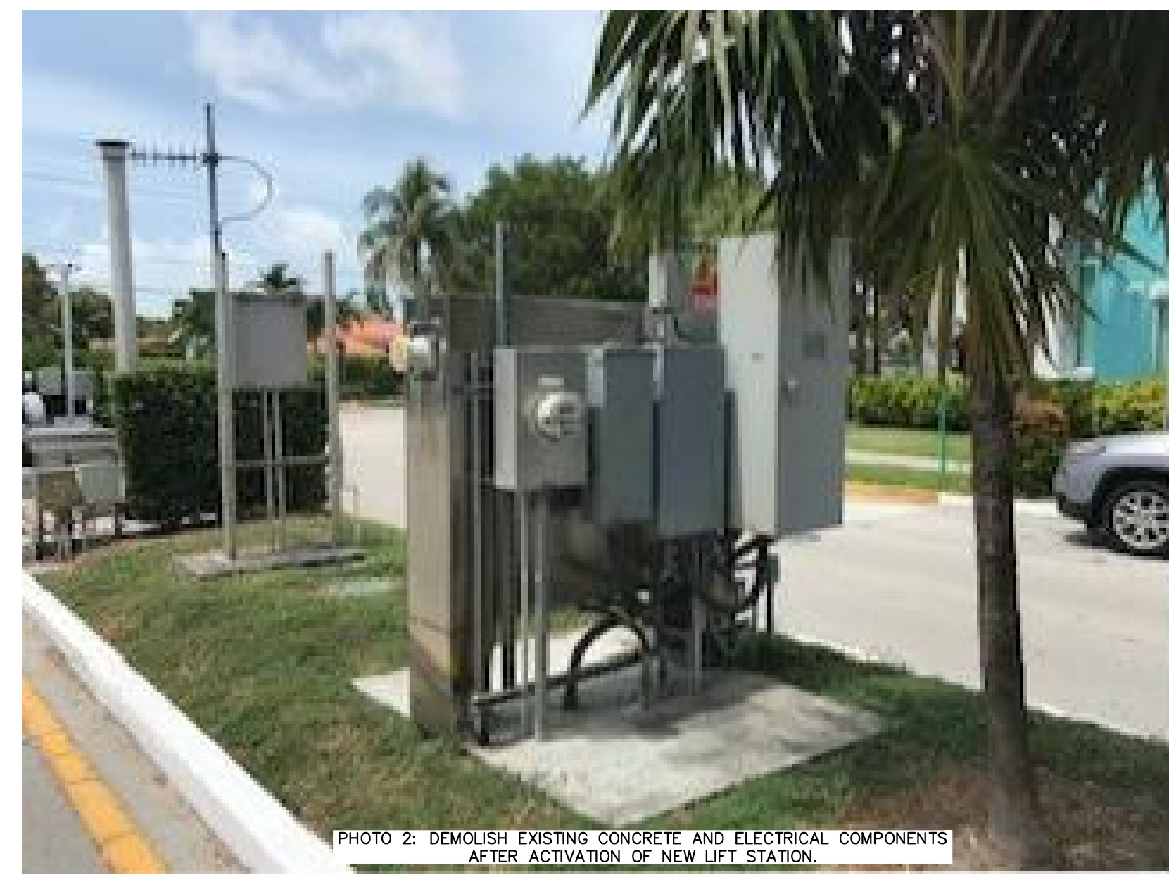
PHOTO 2: DEMOLISH EXISTING CONCRETE AND ELECTRICAL COMPONENTS AFTER ACTIVATION OF NEW LIFT STATION.
