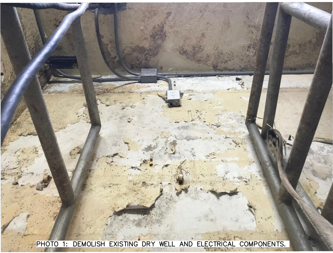
PHOTO 1: DEMOLISH EXISTING DRY WELL AND ELECTRICAL COMPONENTS.
