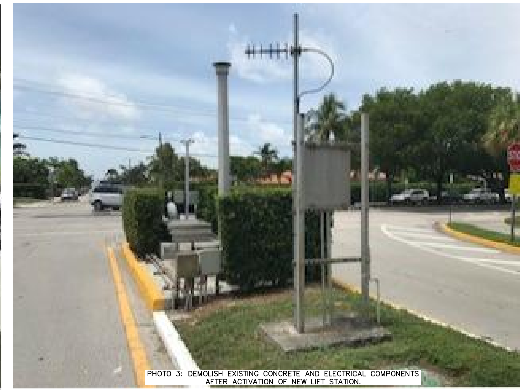
PHOTO 3: DEMOLISH EXISTING CONCRETE AND ELECTRICAL COMPONENTS AFTER ACTIVATION OF NEW LIFT STATION.
