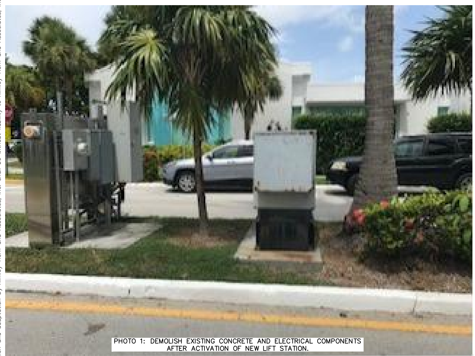
PHOTO 1: DEMOLISH EXISTING CONCRETE AND ELECTRICAL COMPONENTS AFTER ACTIVATION OF NEW LIFT STATION.
