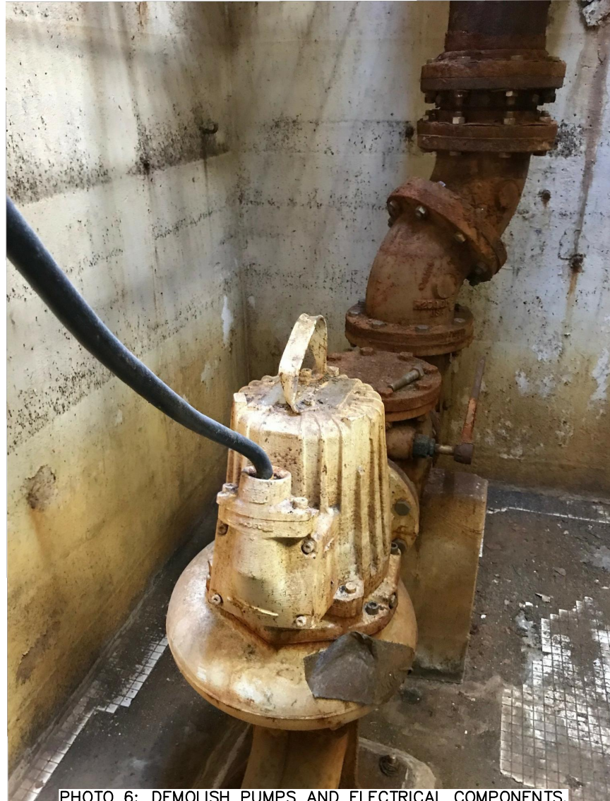
PHOTO 6: DEMOLISH PUMPS AND ELECTRICAL COMPONENTS.
